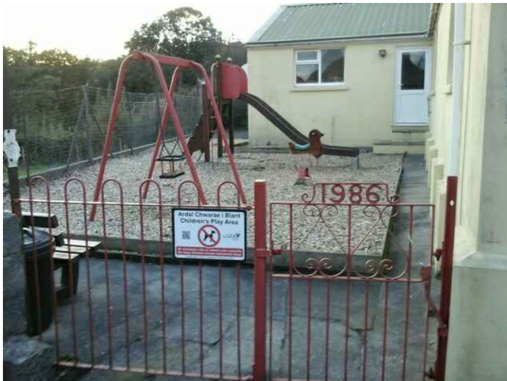
Y Parc cyn y prosiect / The Park prior to the project
